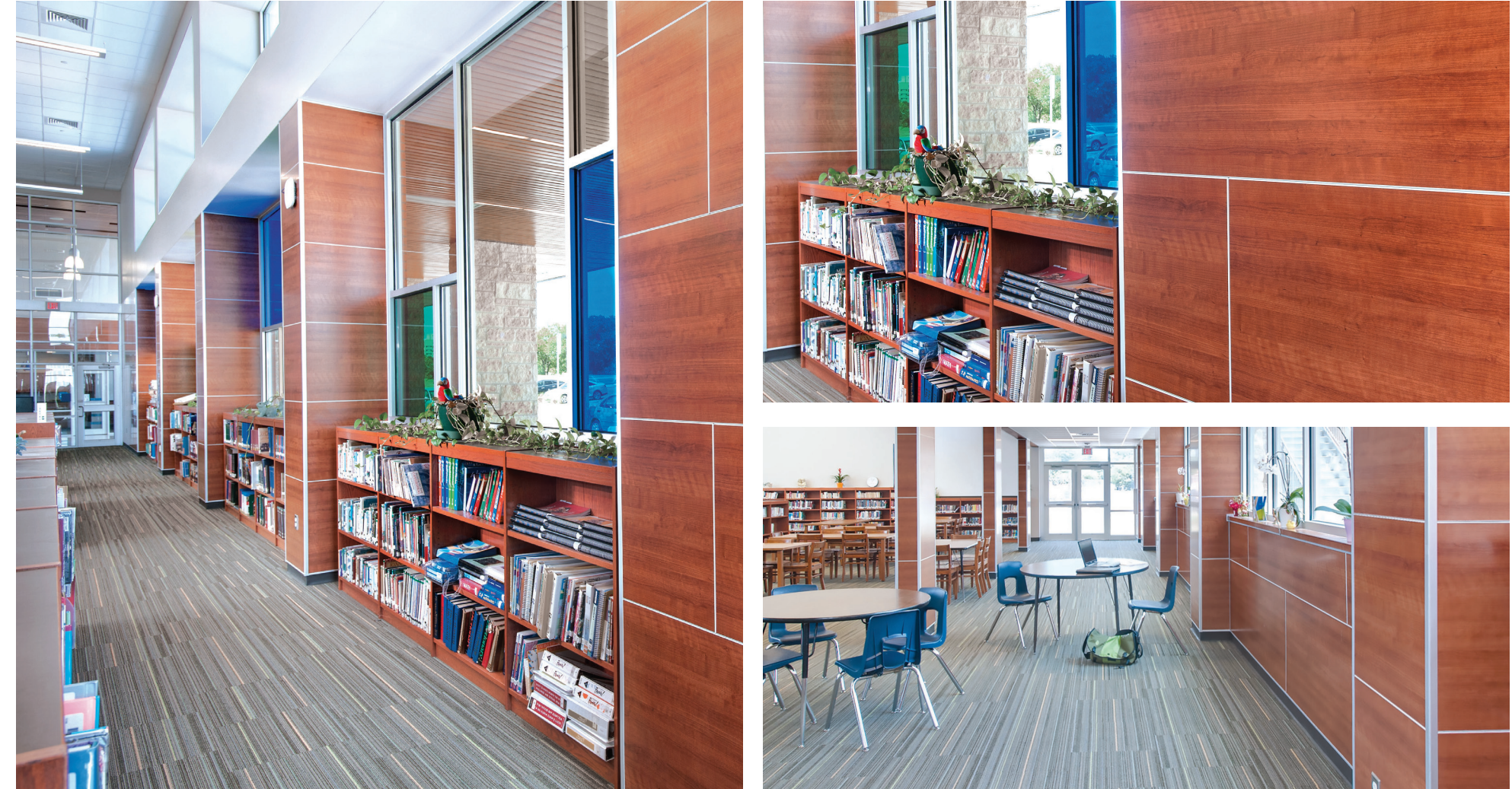
Horizontal panel orientation with a woodgrain pattern HPL panel surface and a 3mm platinum color edge banding featuring a hidden divider molding (302) to create a framed modular look.
