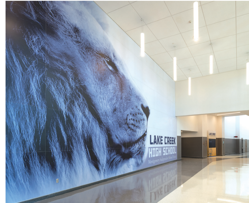
Horizontally oriented 4'x10' custom laminate panels with a 1/16" wide clear anodized reveal moldings.
