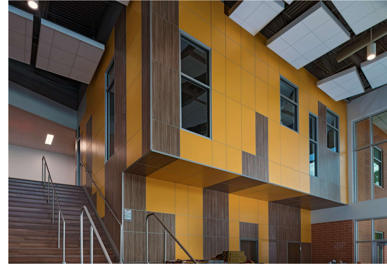
HPL panels with a 1/4" wide divider molding. Extensive field dimension work was required to match the various window sizes with the panels to get everything to align. Many different panel sizes were required, resulting in a more expensive, but well worth-it installation.
