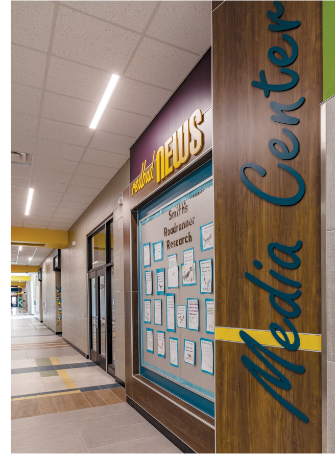
Variety of different HPL patterns and colors are all brought together in the same system with a 1/4" wide reveal between panels.
