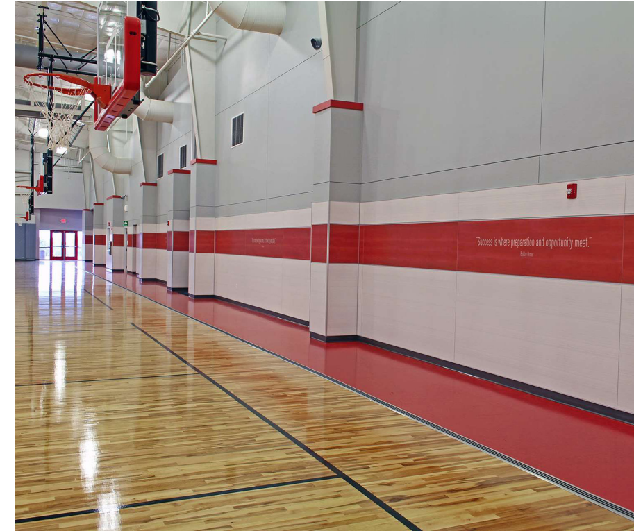
Vertical molding with a 1/16" wide reveal divider molding. Horizontal panel divider molding is 312 channel molding. This creates a strong horizontal banding appearance and minimalistic vertical seams.
