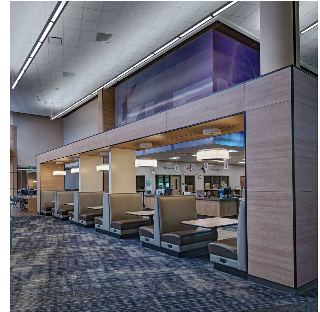
Banquet seating features woodgrain HPL surface with a 1/16" black divider molding reveal.
