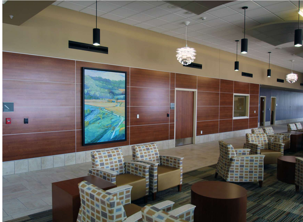
Resembling a tile grout line, the ¼" wide concave profile divider molding is easy to clean. Paired with HPL panels for durability and ease of maintenance.
