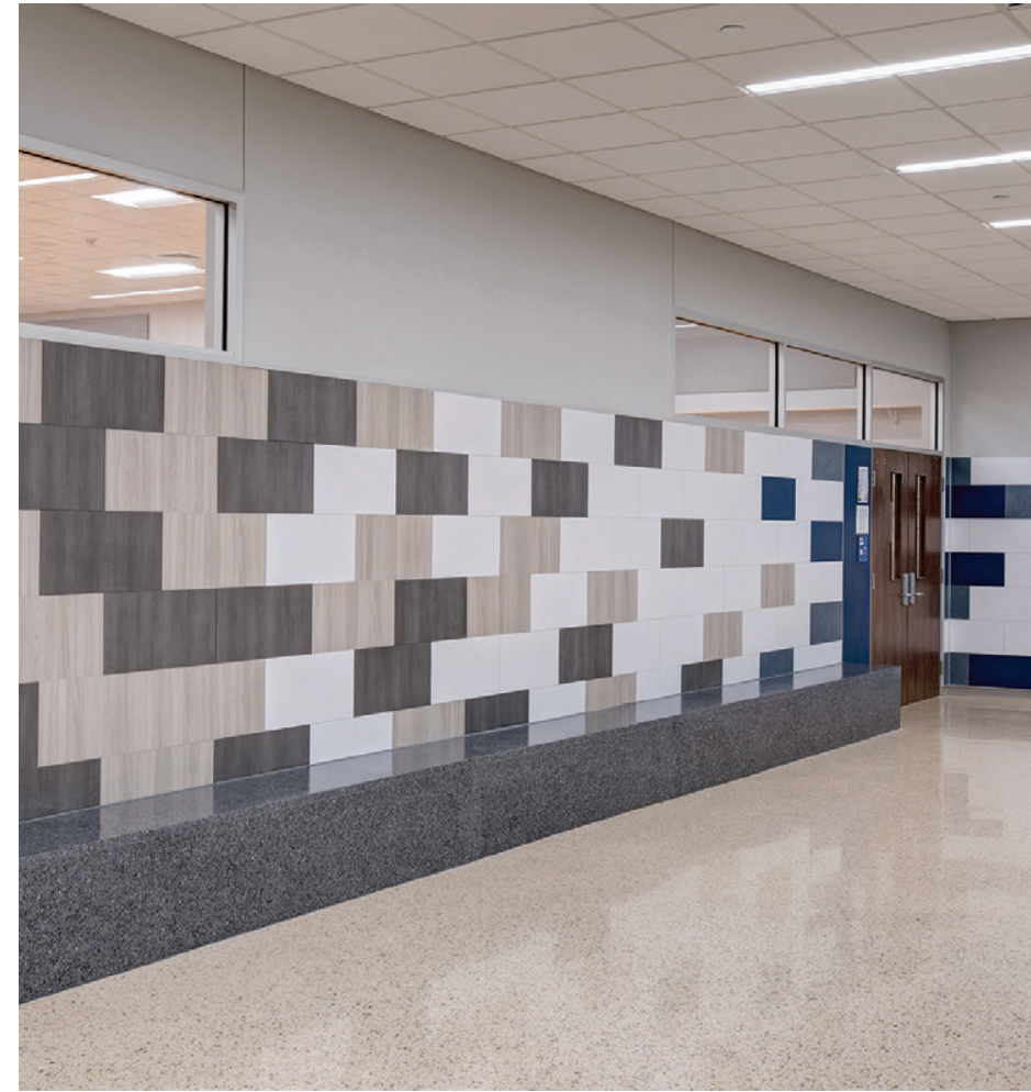
A 1/16" wide molding reveal minimizes the joints between the different color panels.
