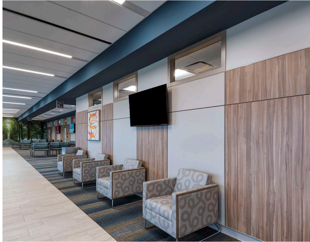
HPL surfaces will stand up to the various healthcare cleaning solutions used in hospital environments. Shown in a clinic lobby with a 1/4" wide divider molding paired with HPL panels.
